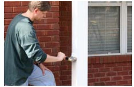
**10.** Prime with an oil-based primer and paint immediately. You can also stain YellaWood® columns with an oil-based stain with water-repellent.
