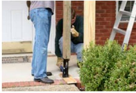
**8.** After ensuring that the column supports the load and is stable, remove temporary support.
